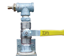
Emergency Control Valve in the 'off' position
