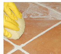
When thoroughly dry remove any remaining grout residues with LTP Grout Stain Remover.
