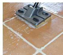
Wash surface with the solution. Do not rinse.
