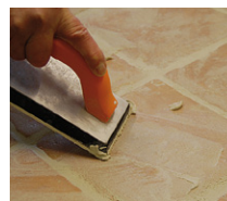
After 1 hour drying time grout the joints.
