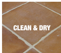
Surfaces must be clean and dry. Under floor heating must be off.
