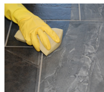
Apply solution to the surface with a mop or sponge Under floor heating must be off.
