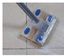
Mop the surface of the tiles and grout joints with the solution. Do not rinse.
