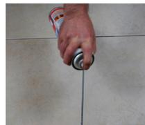
Spray 15-20cm from the surface along the grout joint.
