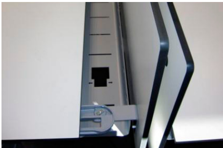
Access to wiring using a movable table top
