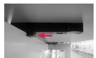
Security Blockage Device
